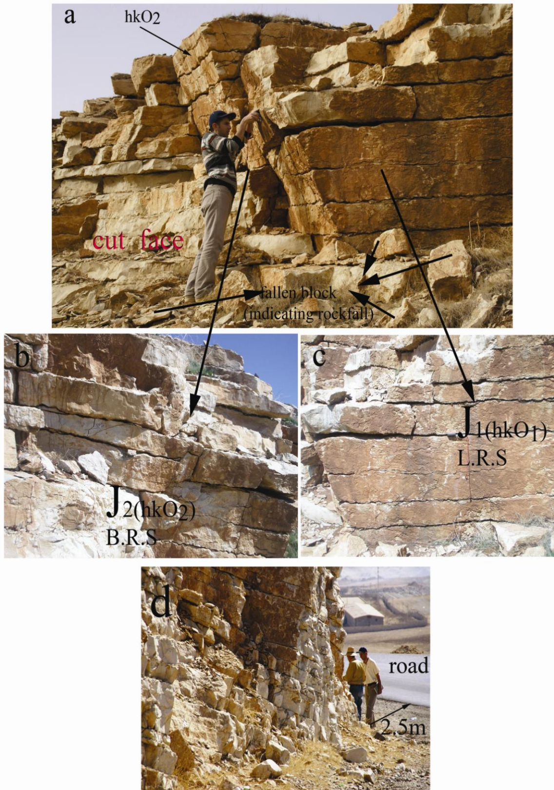
Plate (4-14):a) Lateral view of the slope at station No.9 on the main road shows cut face and fallen rocks b) Shows joints of J_2(hkO_2) B.R.S) (c)Shows joints of J_1(L.R.S) (d) Lateral view of the slope at station No.9 shows the main road from Dokan to Khalakan
