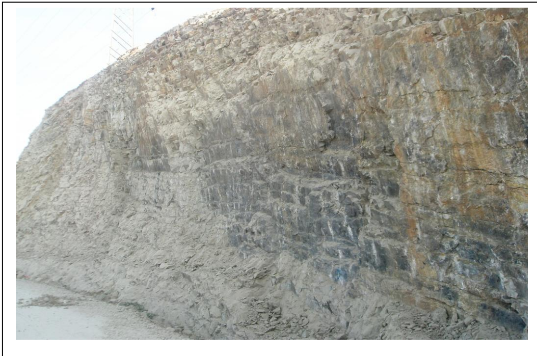
Plate (4-1): b) Unstable slope after cutting its toe at station No.1
