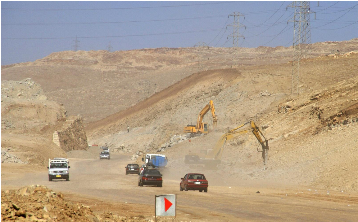
plate (4-7d): The processes of widening of the road between Dokan to Khalakan at station No.4
