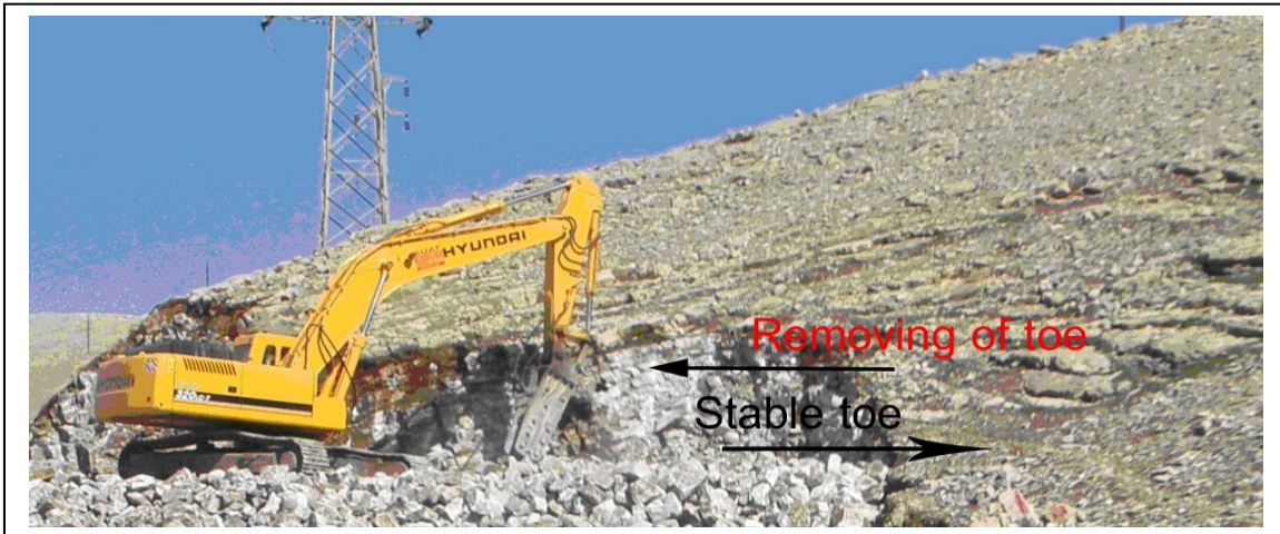
Plate (4.1): a) Shows the process of destabilization at station No.1 due to road widening and removal of the toe
