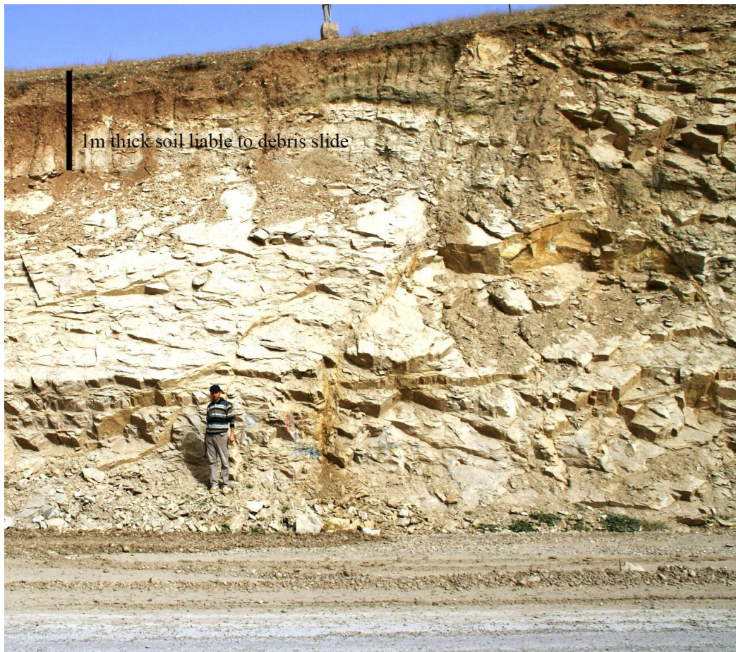
Plate (4-3): Frontal view of slope at station No.2
