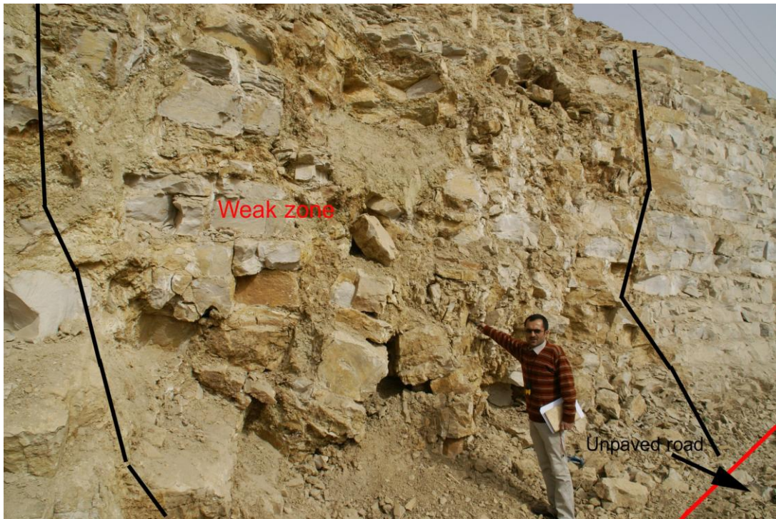
Plate 4-10a: Shows large weak zone at station No.6
