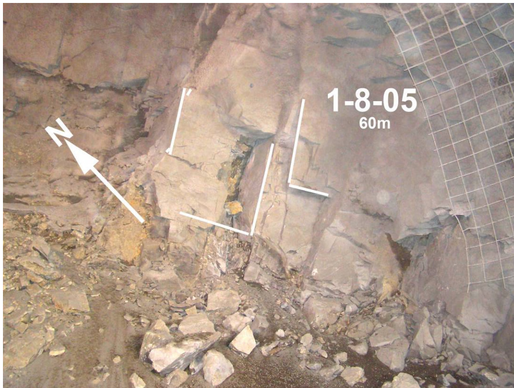
Joint analysis of the tunnel for expecting of the rockfall inside the tunnel at length of 60m from the inlet ( southwestern end
